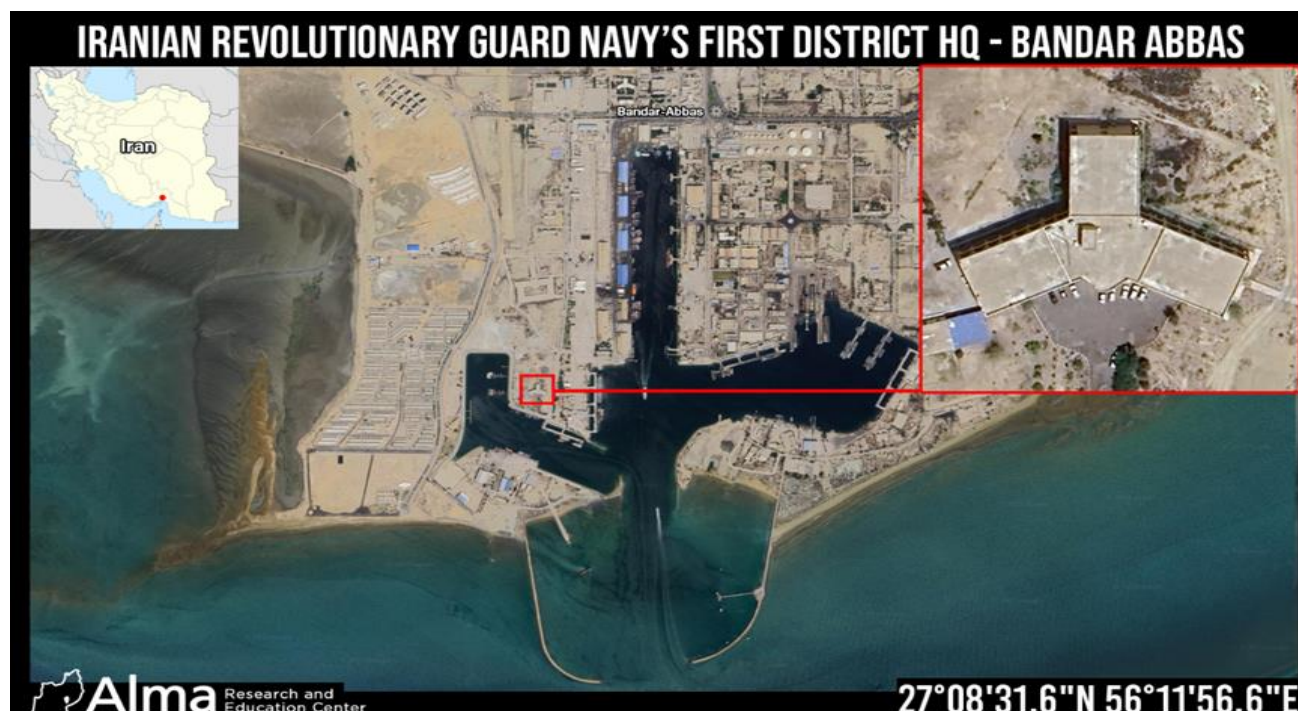
Above: 1 st . Naval District Head Quarters
